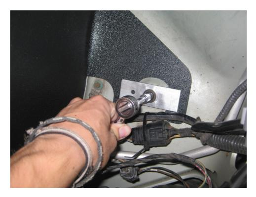
The enclosure should also be mounted at the top using the existing outer hole in the bodywork and the L-shaped bracket provided.
