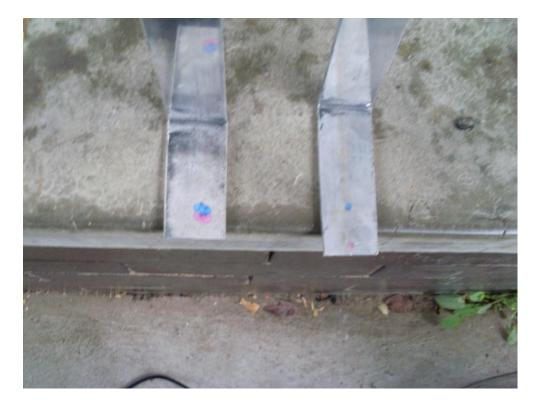
The holes which are drilled will use the 5mm self-tapping screws to secure the bracket to the reo bar.
