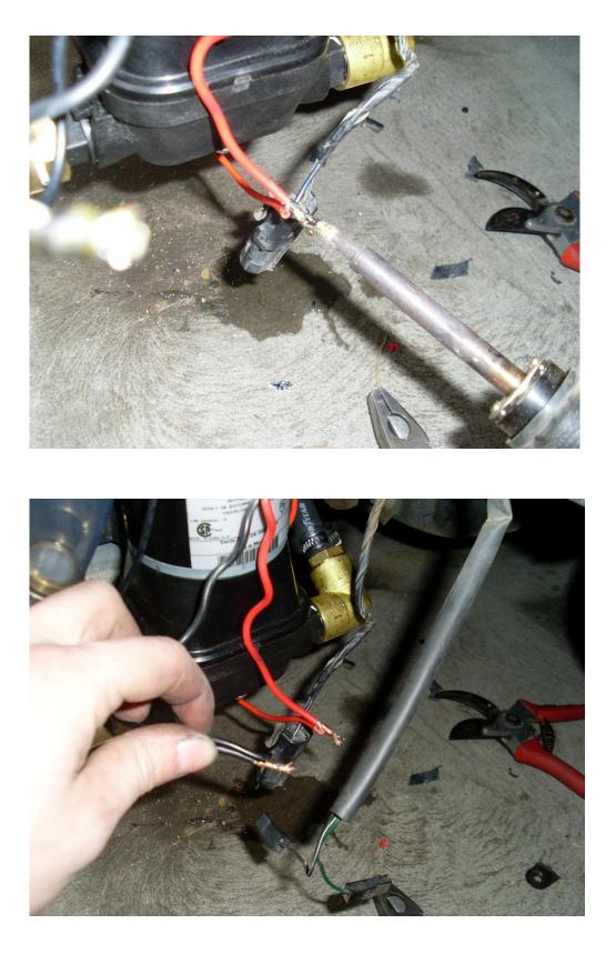
Ground the negative pump wire to the battery using an eyelet electrical connector.
